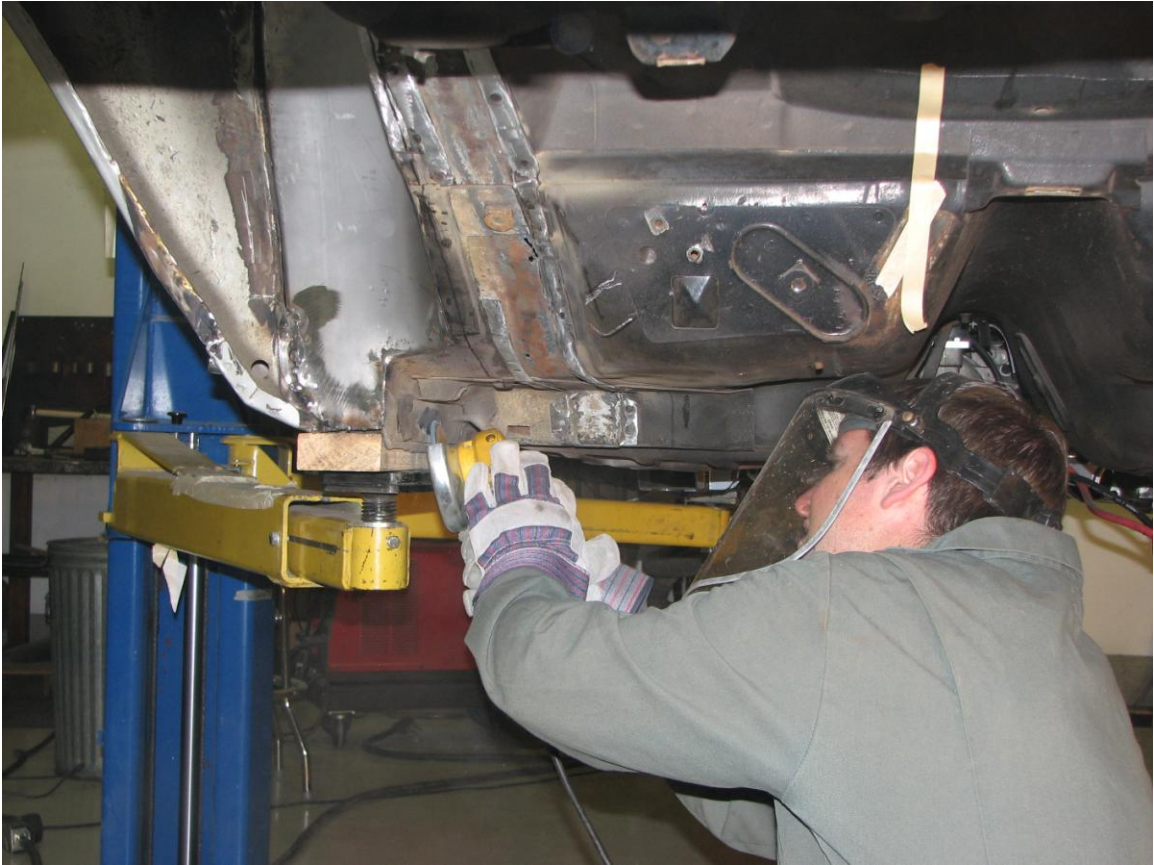
(Photo 4) Preparation for Welding: Here the crossmember-to-pinchweld weld area is being cleaned with a fine disc.
