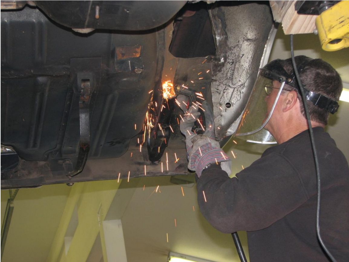
(Photo 1) Rail Removal: In this example, the frame rail is cut at the top radius using a plasma cutter. The remaining vertical section of the rail is then ground flush to the spot-welded strip using a 36-grit disc.
